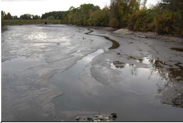
Looking upstream (west) of the dam site on September 25, 2010. The gradual drop in pond elevation had allowed a meandering channel to form.
