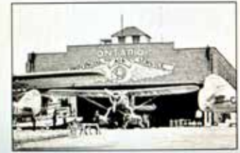
The newly constructed waterfront hanger in Sault Ste. Marie circa 1924.
